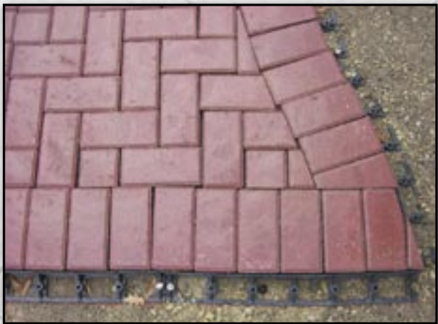
EDGING E Manufacturer's recommended spike spacing.
