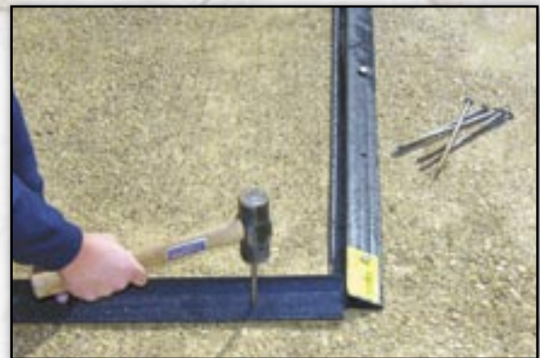
Spiking spaced according to Test Recommended Spacing.
