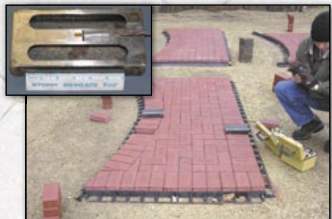
Installation of load sensing steel pavers.
