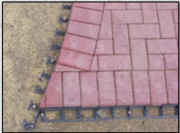
EDGING E Test recommended spike spacing.
